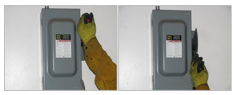
Switch off the grinder's breaker box before performing any maintenance on the machine.
