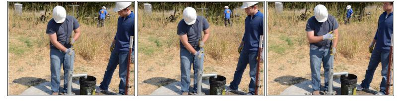
Use the T-handle to push the riser main back down into the well.
