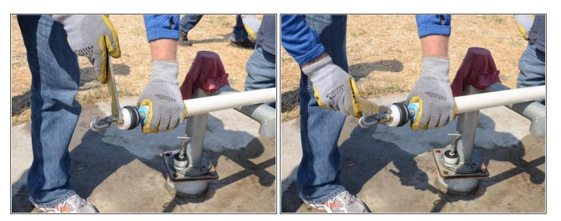
While holding onto the pump rod, use a Tara tool to loosen the jam nut from the hook.
