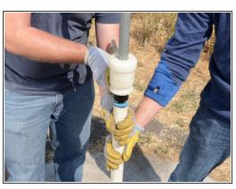
Loosen the jam nut beneath the pump handle using the Tara tool.
