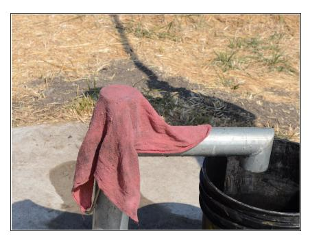
Once the riser main and valves have been removed from the well, place a rag over the top to prevent accidentally dropping anything down the well.
