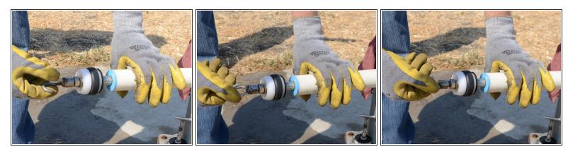
• Unscrew and remove the hook from the base of the pump rod.
