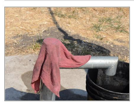
Once the riser main and valves have been removed from the well, place a rag over the top to prevent accidentally dropping anything down the well.
