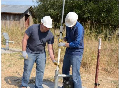
Lift up the handle and riser main until the joint between the two is at a comfortable height to work on.
