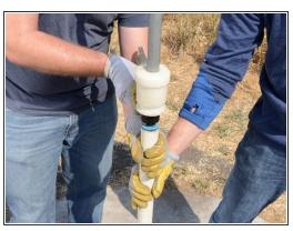
Loosen the jam nut beneath the pump handle using the Tara tool.
