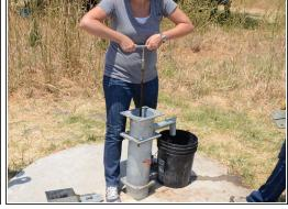
Use the T-handle to pull the pump rod straight up out of the well.
