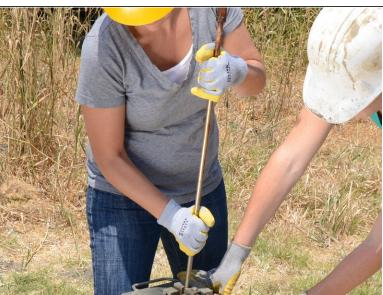
Make sure there is at least 6 inches of space between the joint and the rod clamp to allow yourself enough room to work. If necessary, continue pulling the rod out of the well before tightening the rod clamp to ensure sufficient spacing.
