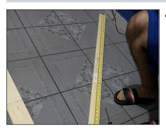
Using your measure tape, measure the old boards and write down the measurements.
