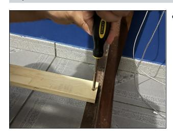
Remove the old boards using the Phillips #1 screwdriver.
