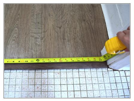
• Measure the exact width of the doorway using a tape measure.
