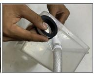
• With a telfon tape properly wrap the soft PVC pipe for no leakage of water.
