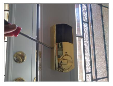
• Using the Phillips #1 screwdriver, remove the three 8 mm screws on the left, right and bottom side of the cover.
