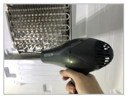
Using a hair dryer or heat gun, melt down any ice buildup in the draining well.
