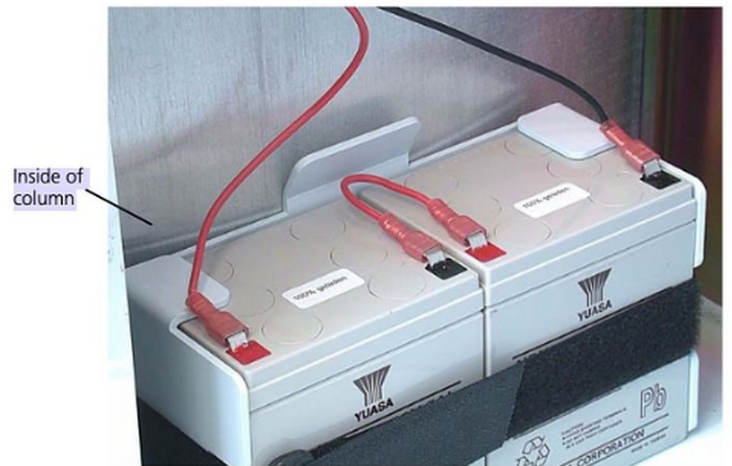
Figure 11-5. The 12 V backup batteries in the column
