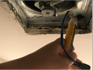
Unplug the unit. Using a circuit tester, confirm that there is no power running through the fan's circuit.
