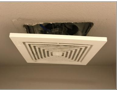
Carefully remove the grill cover on the unit by grasping the outer edges and pulling downward, toward the floor.
