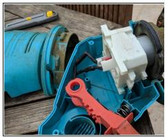
• Remove the 6 screws now visible in the blue part. Open it in two parts.
