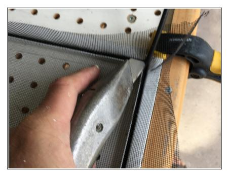
• Use a new sharp blade in your utility knife to cut through pet screen
