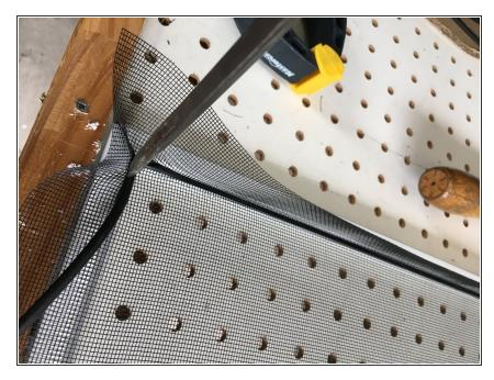
• Get the spline started in one corner by forcing it in with a flat blade screwdriver
