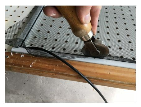
Pre roll the pet screen into the spline groove. Make sure the cloth goes in square and flat. Pull it out and try again if it does not.
