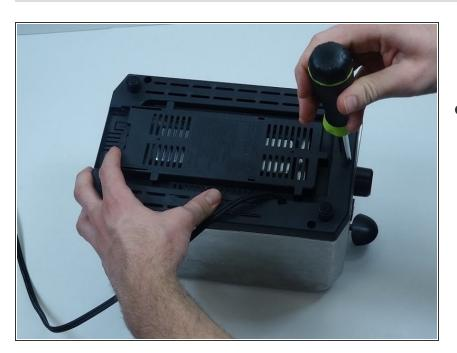
Screw on the bottom of the toaster using all five 5mm Phillips #1 screws.
