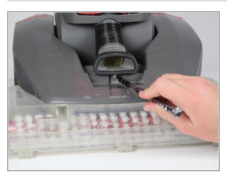
Unscrew the hose by using a Phillips #2 to detach it from the top cover of the cleaner.
